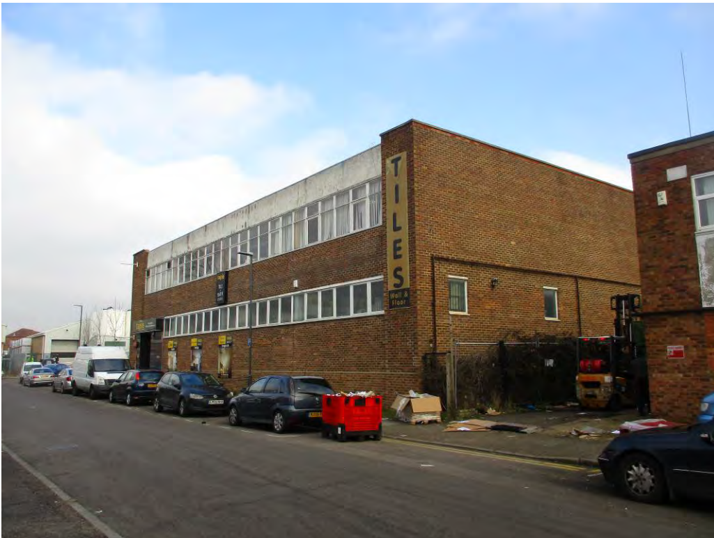
Front (west) elevation facing Brember Road
