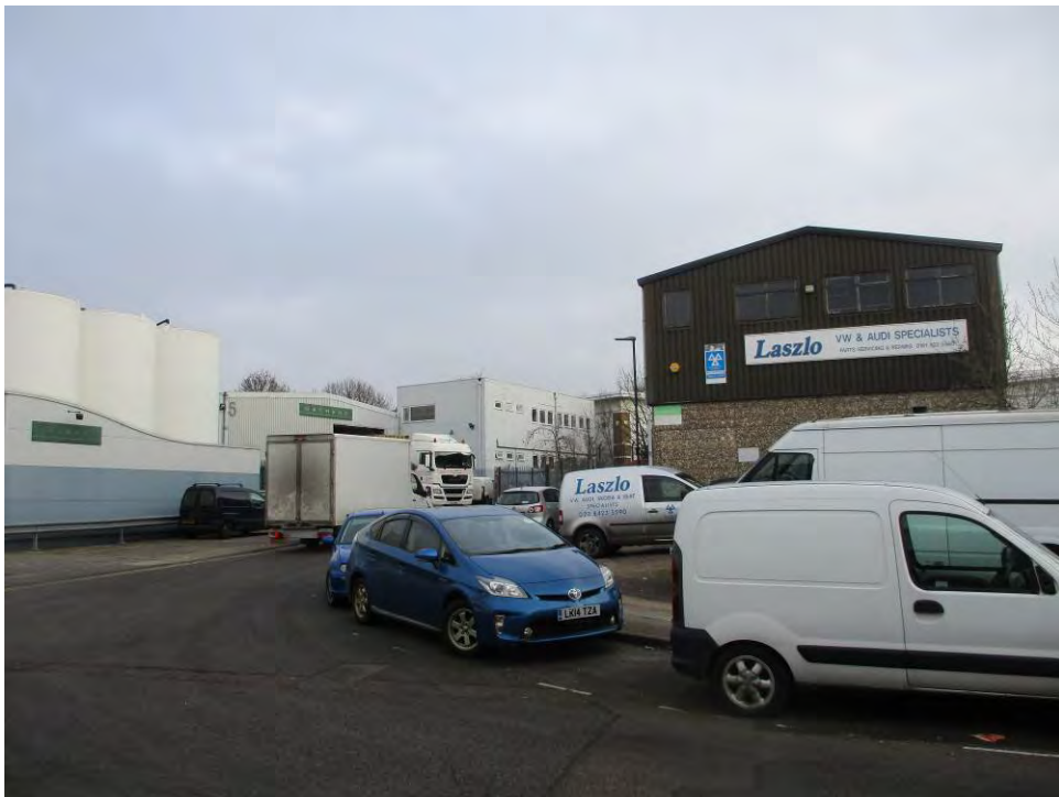
Neighbouring buildings to the north
